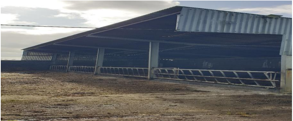
Plate 2.3: Two Bay Slatted Cattle Shed and Associated Slurry Pit for Demolition
