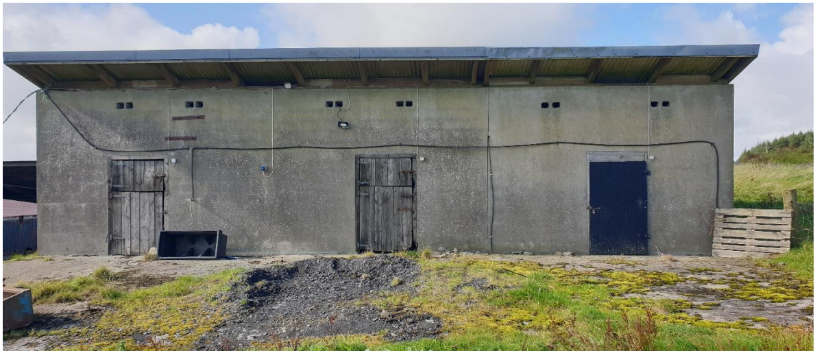
Plate 2.4: Hay Shed for Demolition
