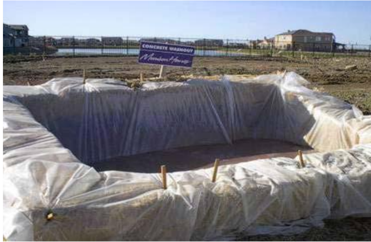
Plate 2.1: Typical Temporary Concrete Washout Area
